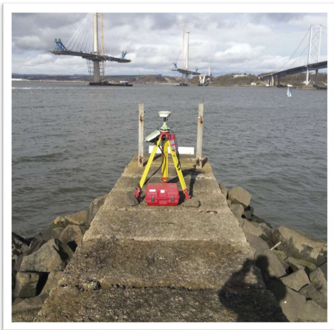
GNSS observations on a pier. Note the new Queensferry Crossing under construction in the background
