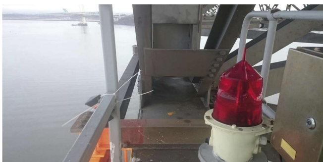
4. The view from the navigation gantry under the Forth Road Bridge, in the background you can see SMB Shackleton who has just sailed from Port Edgar Marina.
