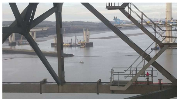
3. The prism reflector installation by 42 Regt RE around port (west) navigation mark on the Forth Road Bridge.
